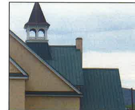
The unique green colored roof of the Oakley City Hall
