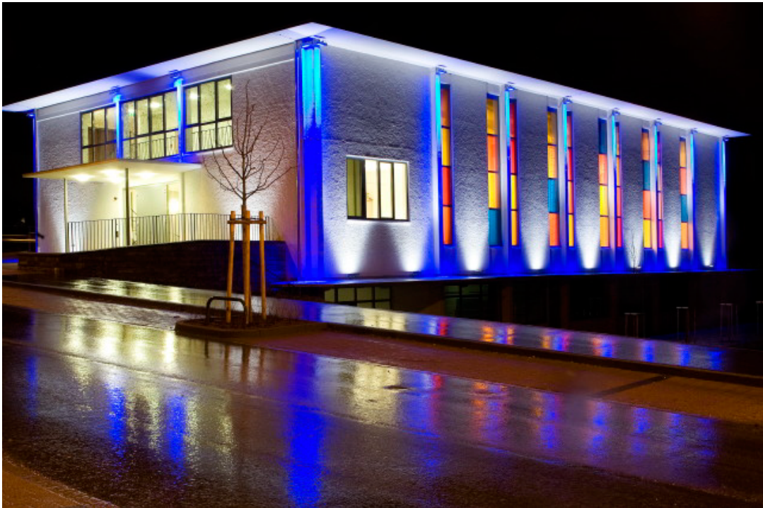
Figure 9-18-6 Example of Poor Architectural Lighting
